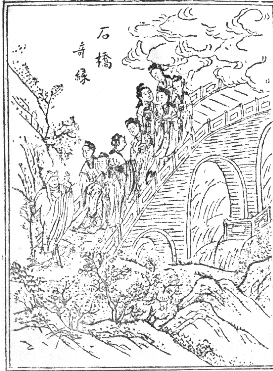
The Fairies on the Bridge
